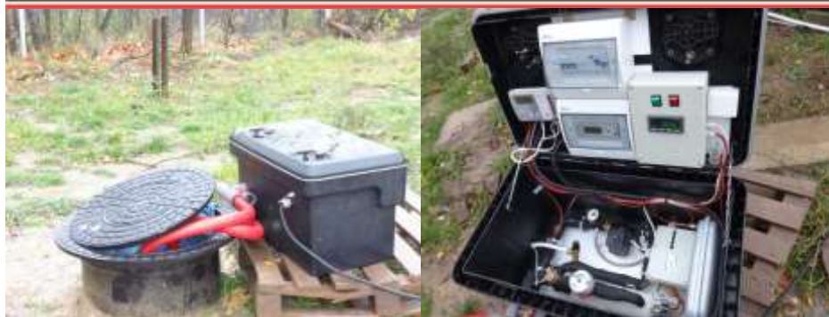
Figure 1. TRT device during borehole heat exchanger testing
